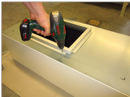
10. Use the four M8 x 25 mm screws supplied to permanently screw down the terminal box to the unit.
