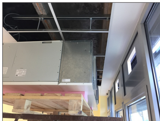
10. Use the four M8 x 25 mm screws supplied to permanently screw down the terminal box to the unit.
